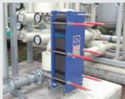
Heat exchanger for exhaust heat recovery
