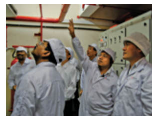
Site inspection in Southeastern Asia
