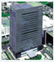
Kyocera headquarters building
